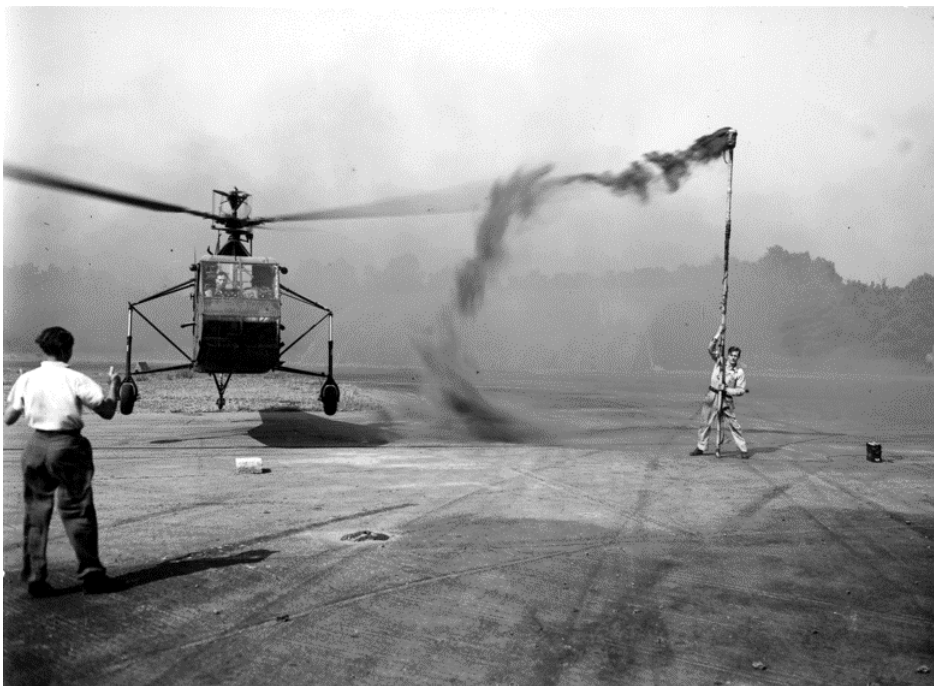
Figure 27. Early experiments in visualising the airflow through and around the rotor disc
